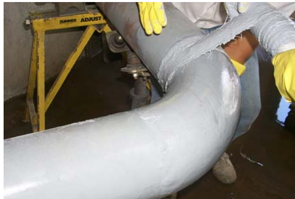
Figure 5 – Repair of pipe elbow fitting using Armor Plate® Pipe Wrap 6-in standard wall elbow with 50% corrosion Unrepaired burst pressure of 4,532 psi • Repaired burst pressure of 6,780 psi
