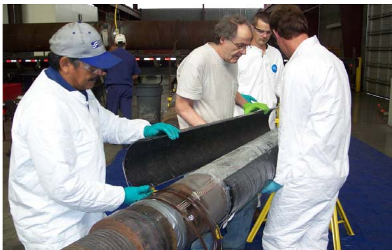
Figure 9 – Installation of the carbon half shells
