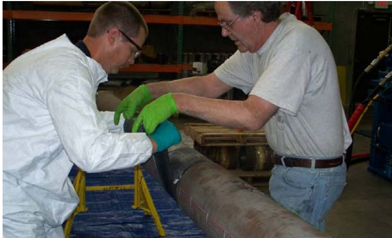
Figure 7 – Installing the hoop wrapped inner carbon layers
