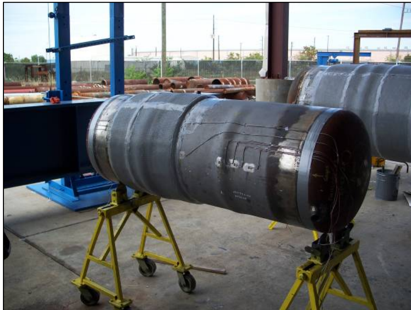
Figure 5 – Photo showing completed installation of Armor Plate ® Pipe Wrap
