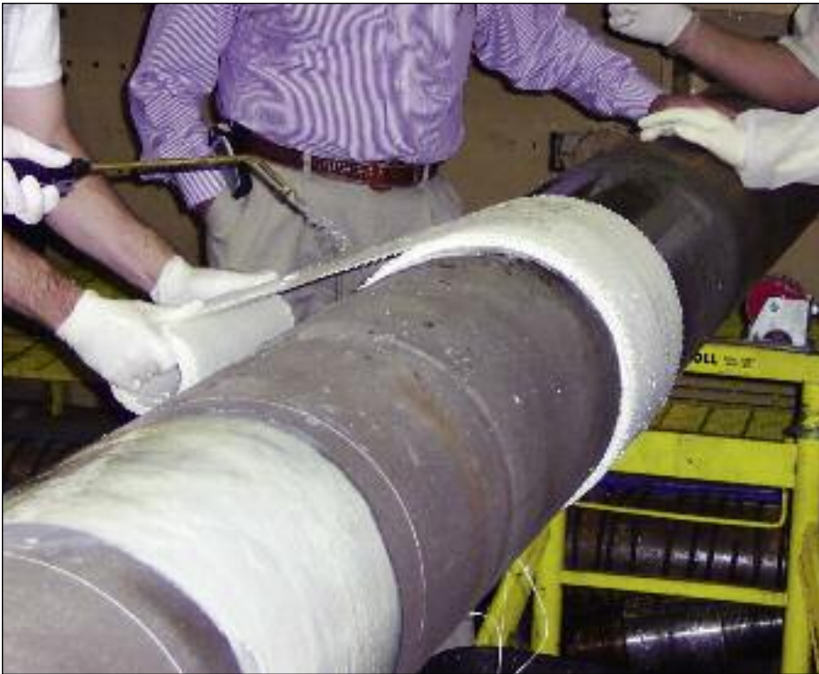
Figure 4. Installing composite material on pipe.
