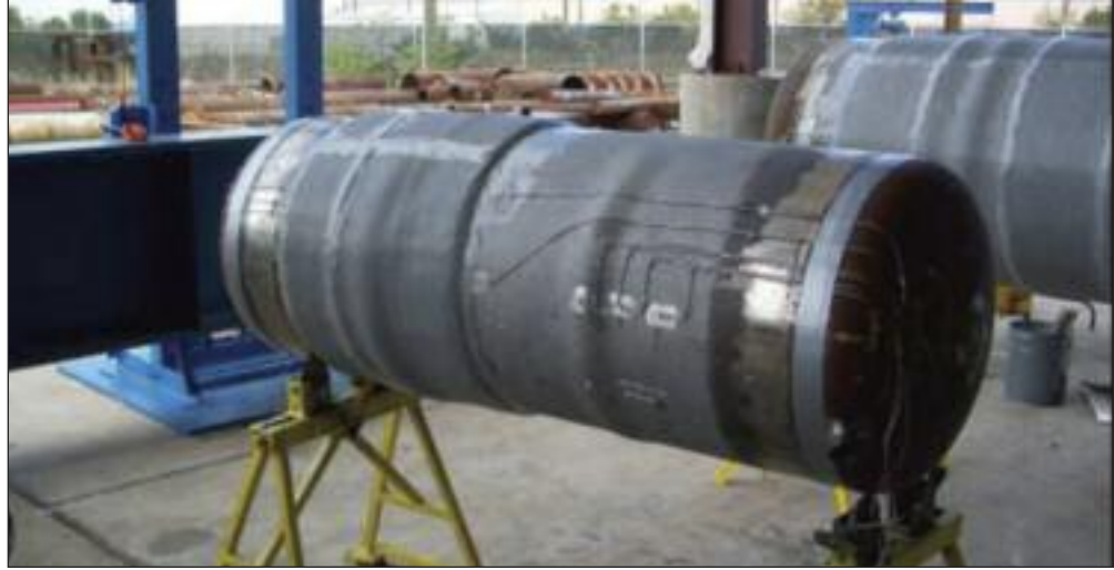
Figure 3. Photo showing completed installation of composite material.
